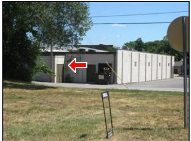
7.1 Picture 6 Store Shed Behind #332
