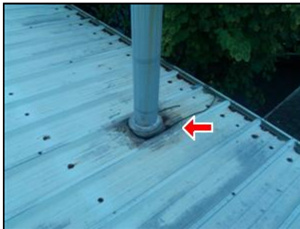
6.0.A Picture 4 Reseal flashings
