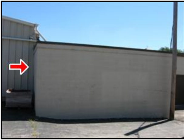
7.1 Picture 7 Back of Store Shed at #332
