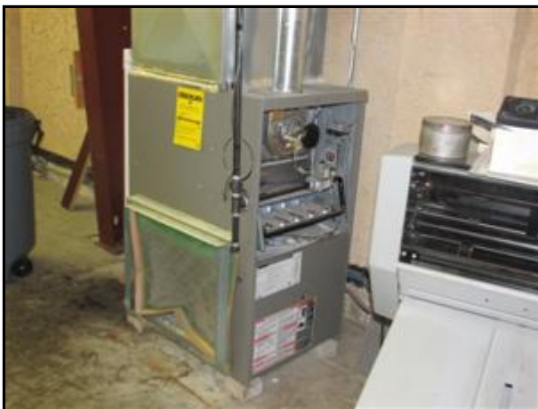
3.1.A Picture 3 South Wall
