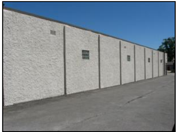
7.1 Picture 4 South Side #332 & Parking Lot
