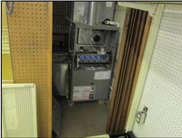
3.1.B Picture 3 South Wall
