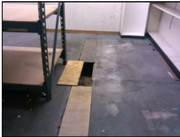
11.6 Picture 1 Trench Drain.
